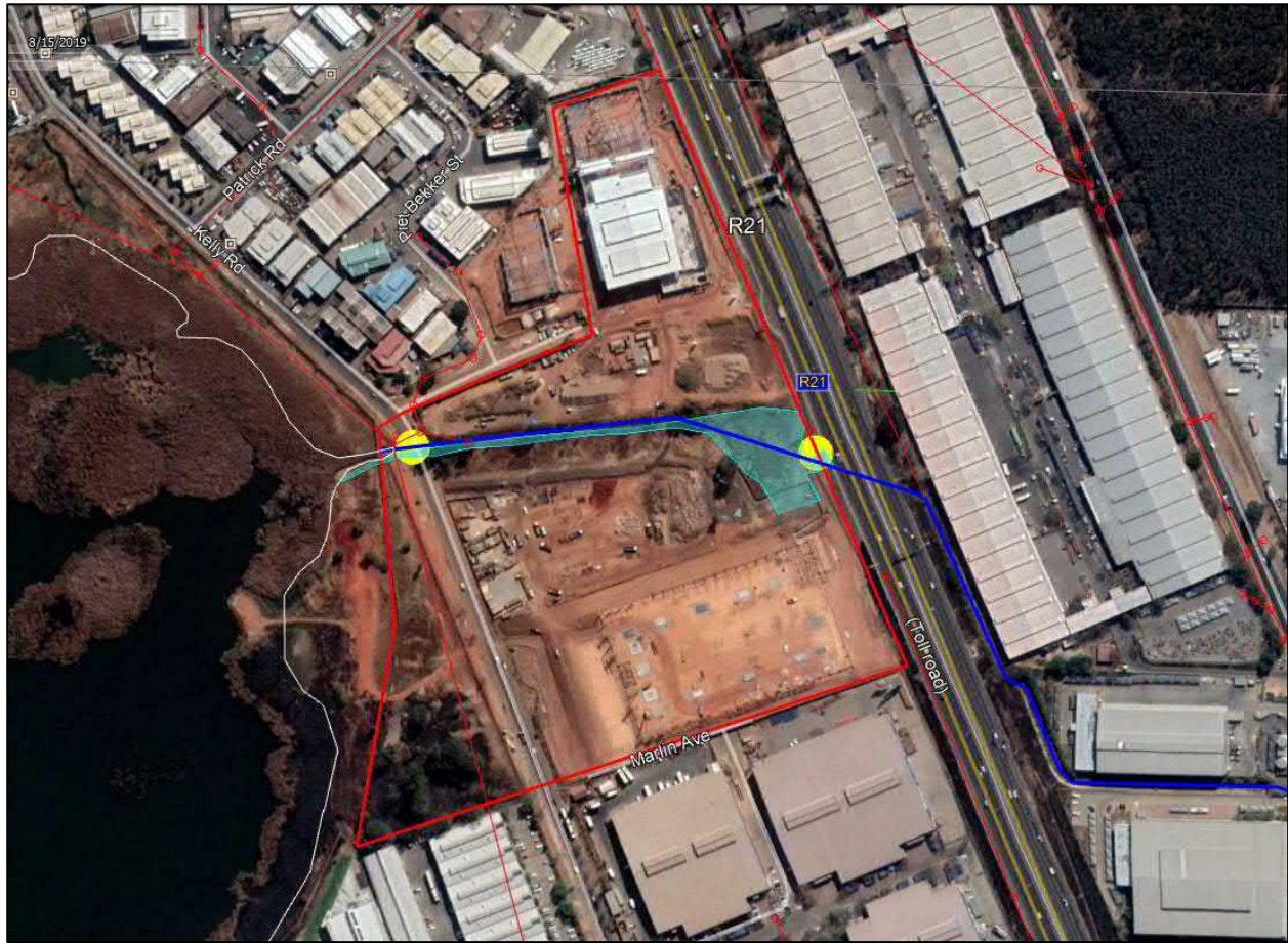
Figure 6: current site conditions (2020)
