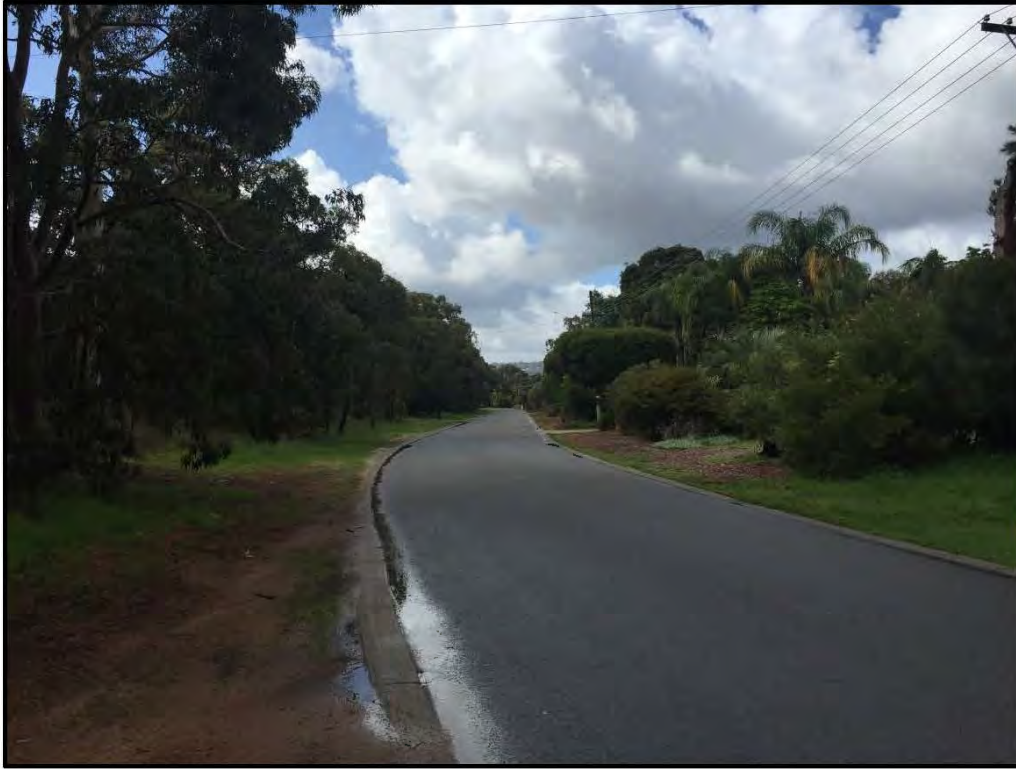
Photo 7: An eastward view along Brae Road
