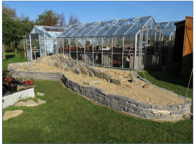
Raised bed filled with sand/grit mix.
