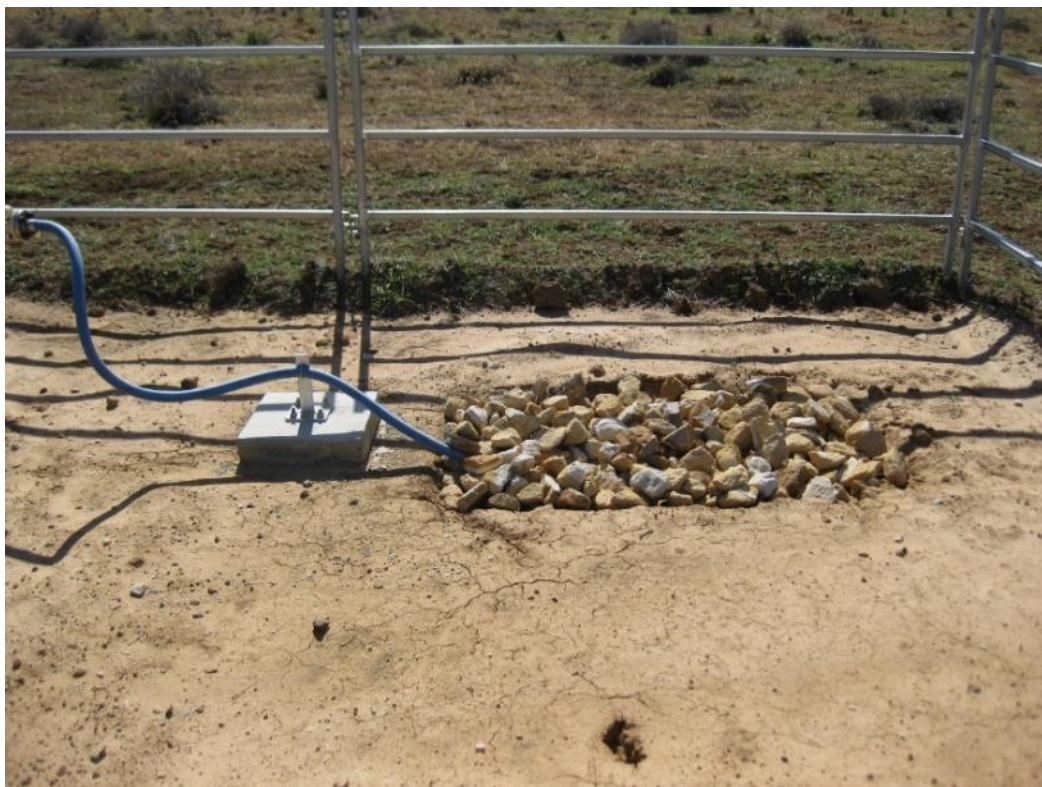
Figure 4 – Example of Current LPD Discharge Design (Single)
