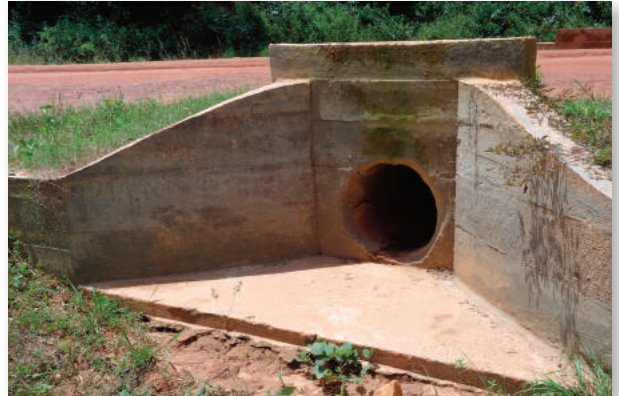
Figure C.6.5 Concrete apron at culvert outlet
