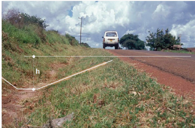
Figure C.2.1: A well-drained pavement
