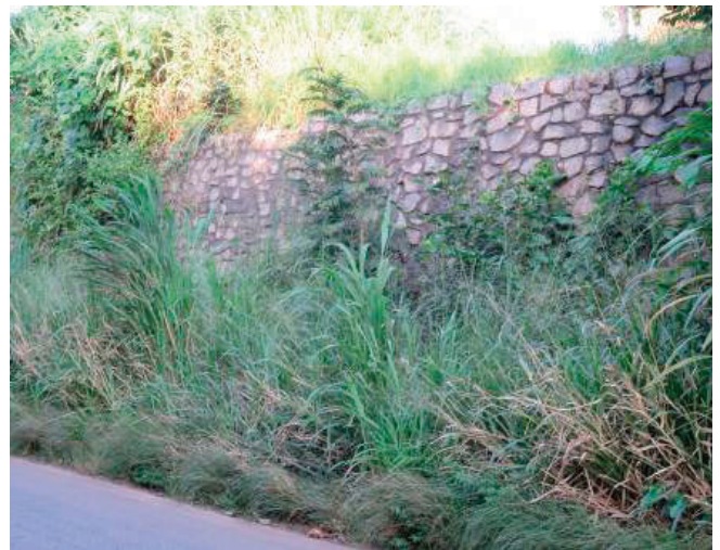
Figure C.7.16 Mortared masonry wall providing shallow support and slope protection
