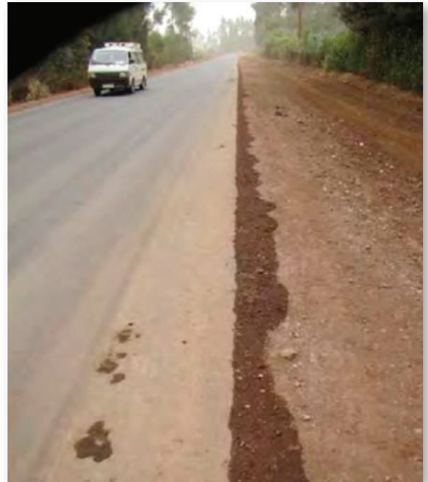
Figure C.2.4 Infiltration of water through a permeable surfacing
