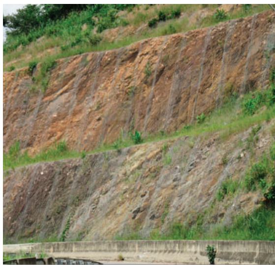
Figure C.7.7 Benched cut slope in rock
