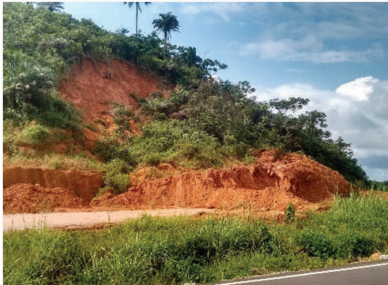
Figure C.7.4 Slope failure in weathered mantle
