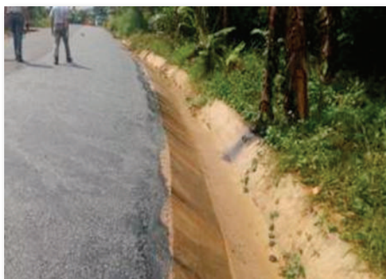
Figure C.4.2 Concrete-lined trapezoidal drain along a sealed LVR in Eastern Region
