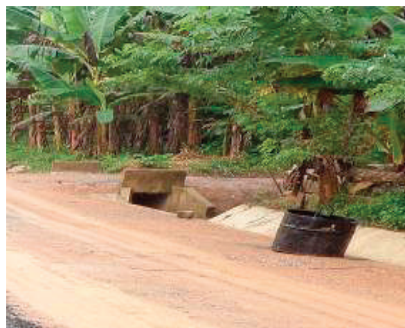
Figure C.4.10 Access culvert at a junction
