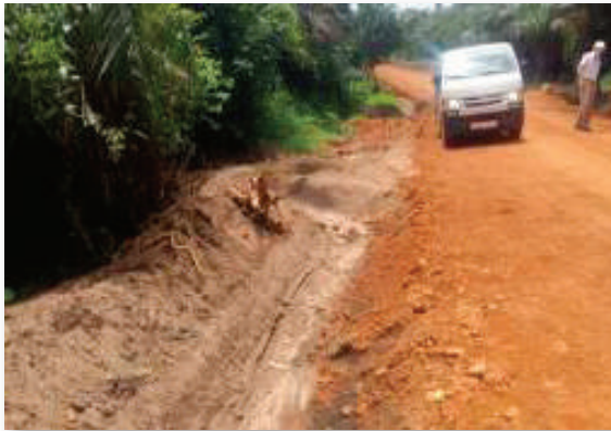
Figure C.4.4 Mitre drain along a LVR
