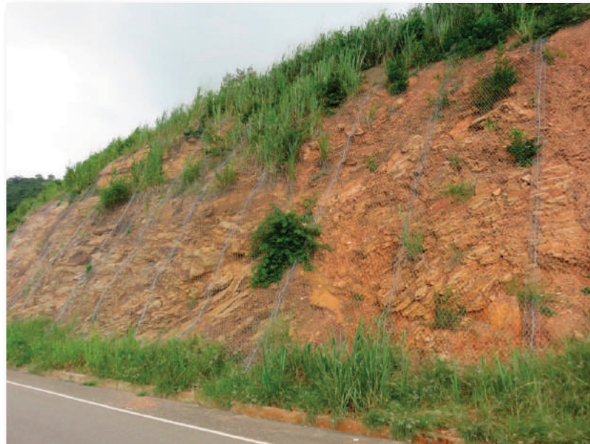
Figure C.7.11 Use of wire netting on cut slope
