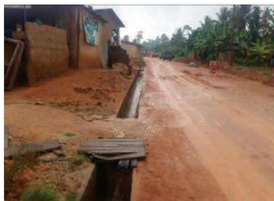
Figure C.4.3 Concrete-lined U-Drain along a gravelled LVR in Eastern Region
