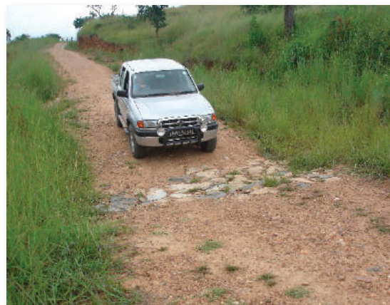
Figure C.4.14 Simple hand packed stone drift
