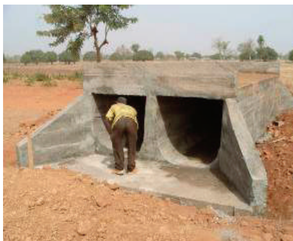
Figure C.4.9 Double U-Culvert
