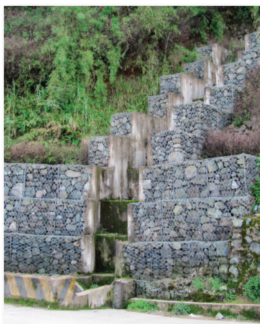
Figure C.6.11 Gabion cascade
