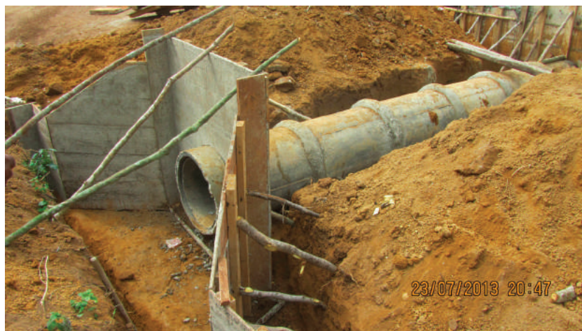
Figure C.6.2 Reinforced concrete pipe culvert
