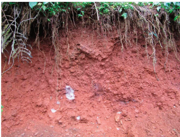
Figure C.7.5 Colluvium/landslide material, vulnerable to failure if cut too steeply
