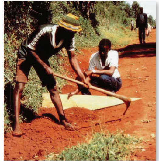
Figure C.8.5 Checking drain shape with template
