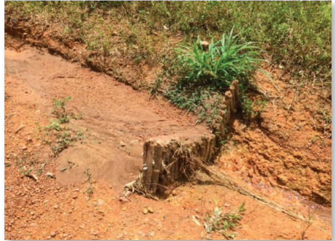
Figure C.6.14 Scour check made from wooden stakes
