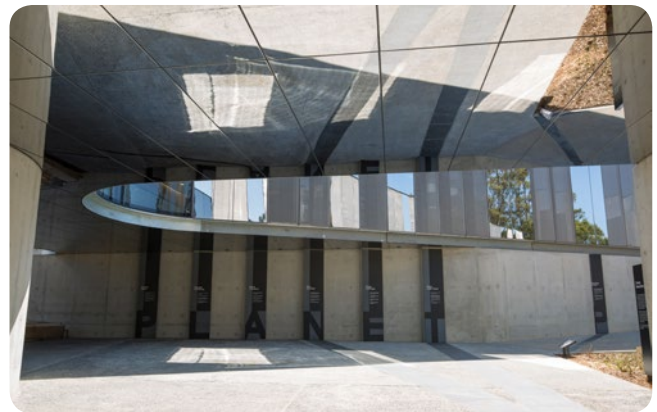
Visitors engage with the work of the building as soon as they enter the surrounding landscape.
