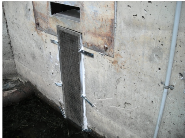
Photograph OS-3. Trash rack after repair.
