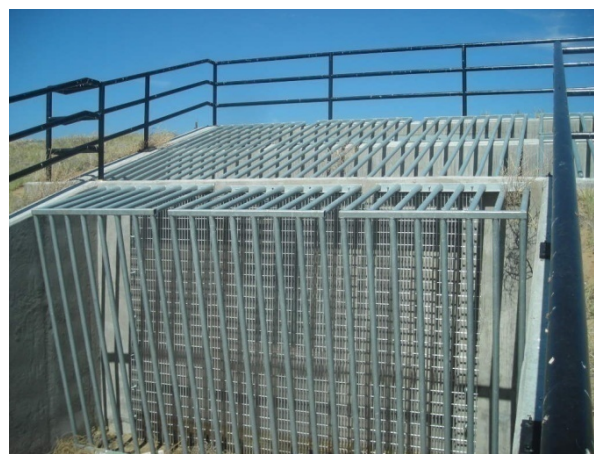
Photograph OS-5. Interruptions in the horizontal members of this trash rack and the spacing of the vertical members allow easier access to clean the water quality grate. A raking tool can be used to scrape the water quality trash rack.
