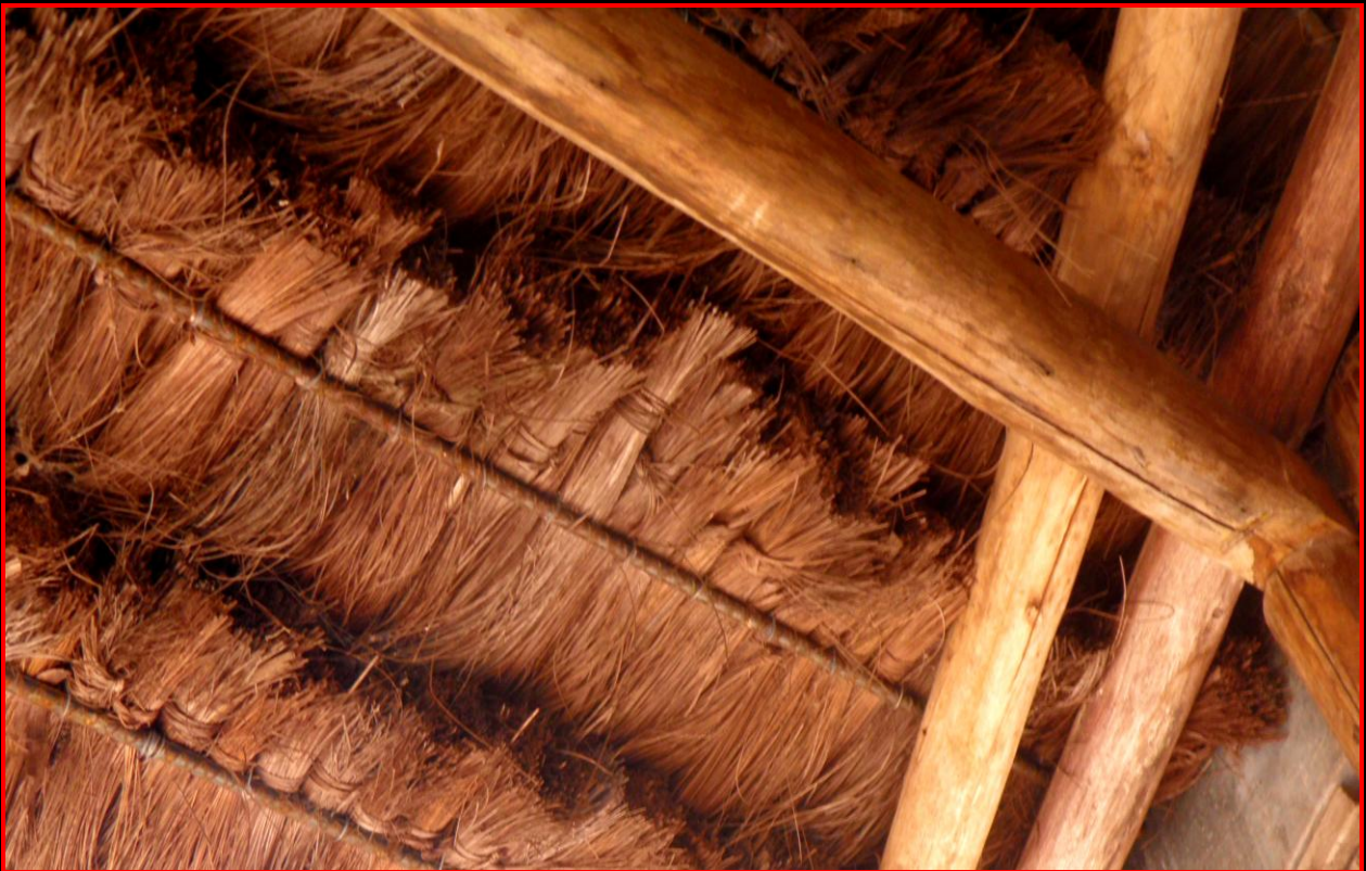
Interior ceiling, Gustavo Heny Airport, Camp Canaima. Photo: Marianela Camacho, 29 June 2012
