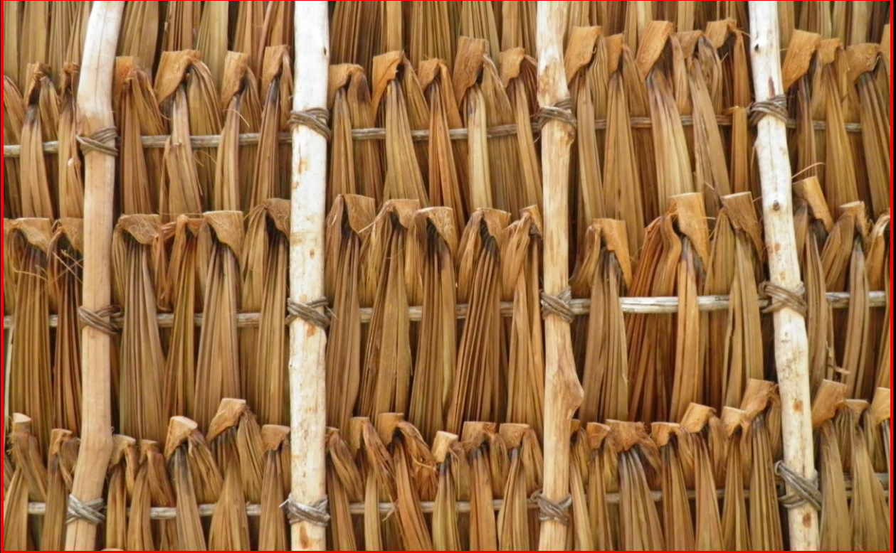
Interior ceiling, Kavac assembly hall construction. Photo: Marianela Camacho, 30 June 2012
