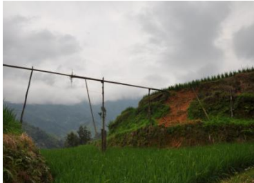
Elevated moso-bamboo water pipeline: use for transporting water on the mountains to the terraces and residents as living water
