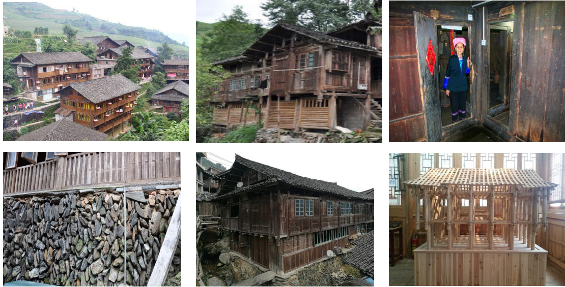
Figure 1-4-19 Traditional architectures in Longji Terraces
