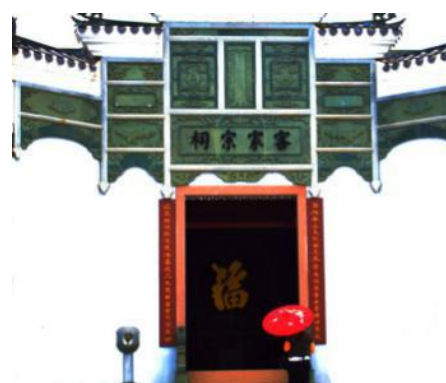
Figure 1-4-42 An ancestral hall of the Hakka in Chongyi
