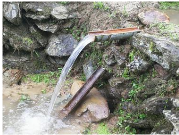
Special bamboo tube: used to buffer the flow momentum, reduce water loss and soil erosion in the places with larger terraced waterfall gap
