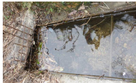
Figure 1-5-21 Grit chamber at the beginning of canals
