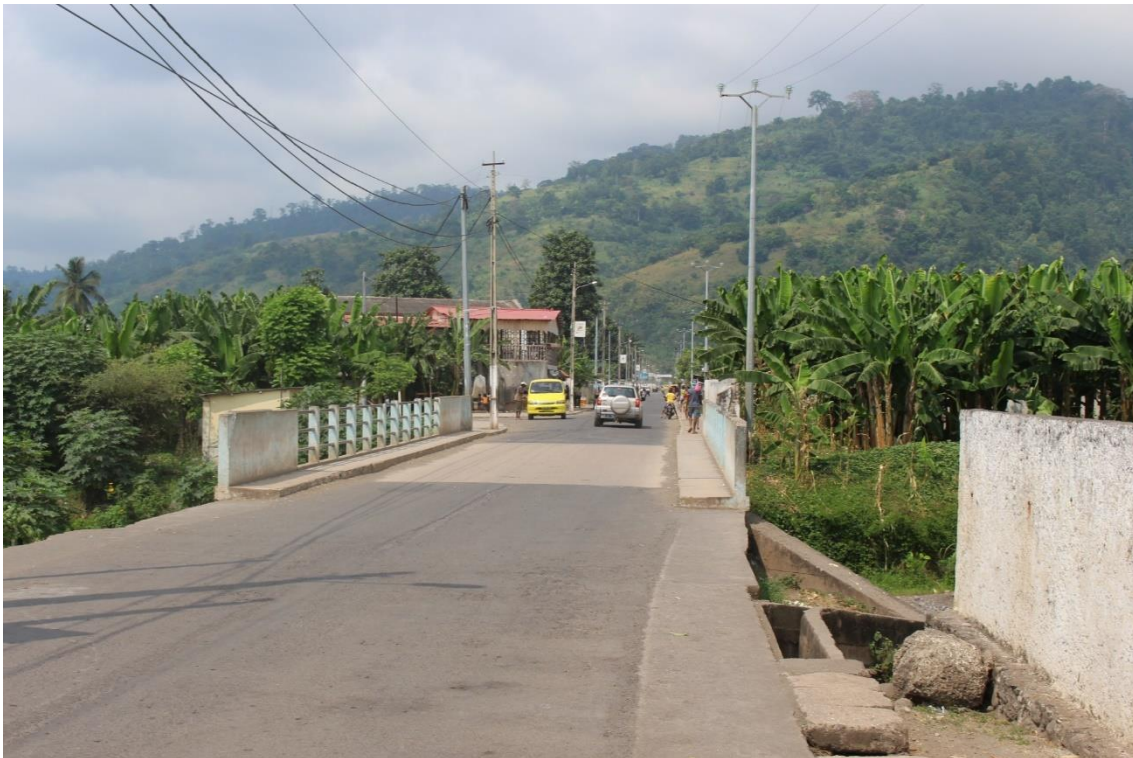
Figure 4-4: A bridge over Provaz river
