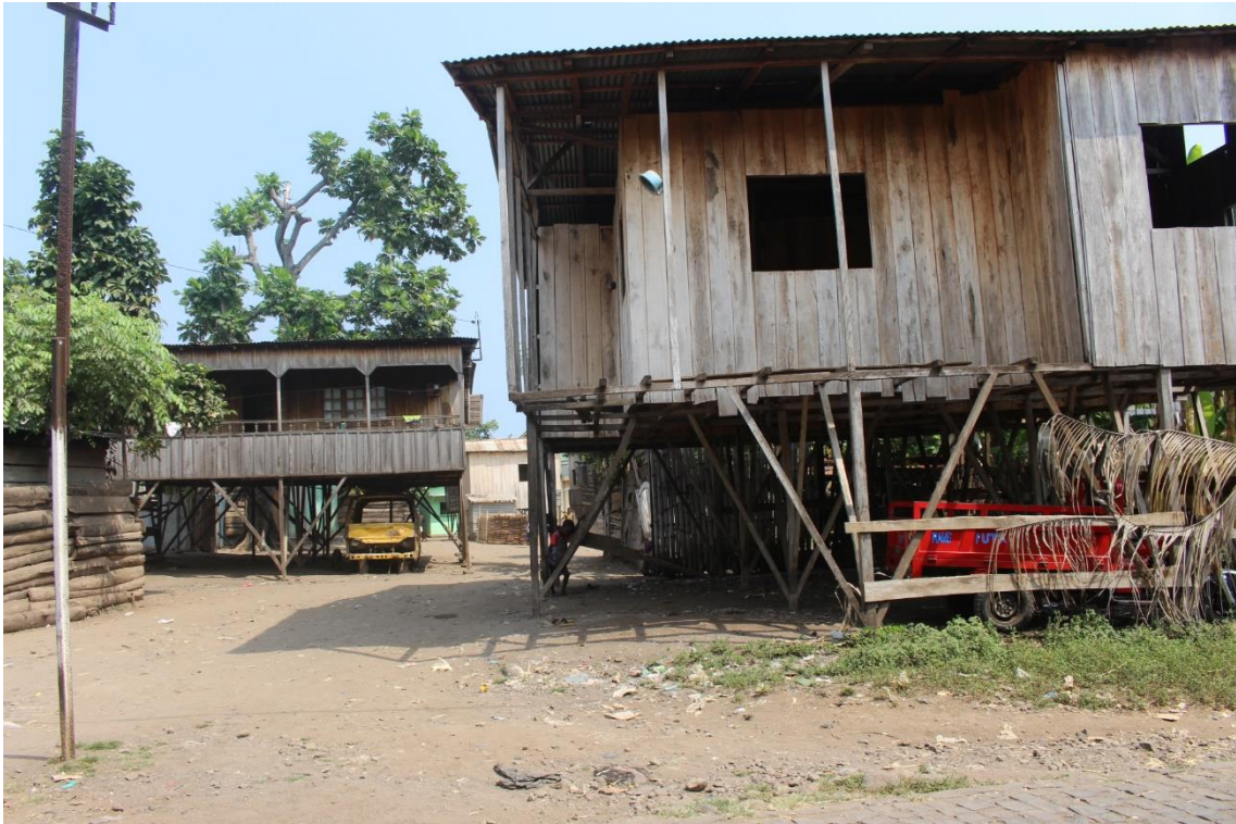
Figure 4-5: Elevated house in Neves for protection against storms
