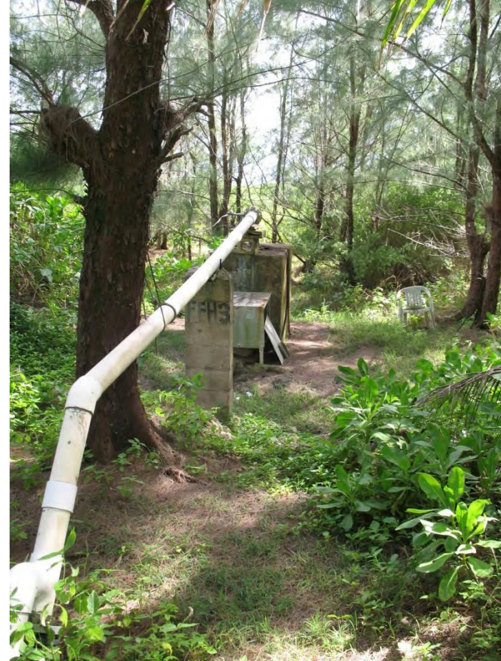
Figure 1-20. Effluent of the Guam Aquaculture Development and Training Center; all water passing through the hatchery is discharged onto open rock and then directly to the ocean. Photograph by S.J. Walsh.
