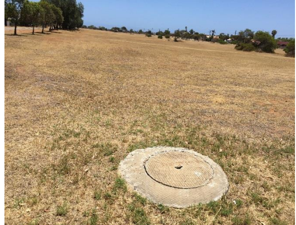
PLATE 8 Sewer inspection pit/lid.
