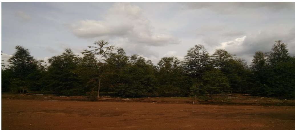
Plate 5: Showing the nursery site under construction and the forest Plantation Site at Royanka
