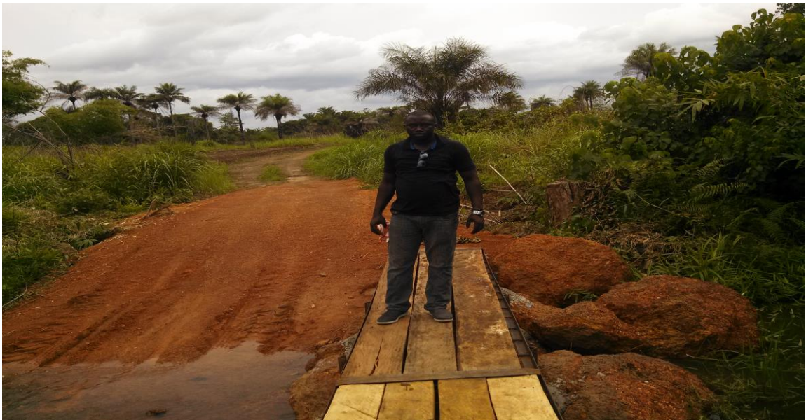
Plate 7: Showing the rehabitated road by Miro Forestry Company (SL) Ltd.
