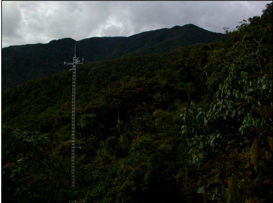
Figure 2.2.2.1: The 40 m leeward forest canopy mast.
