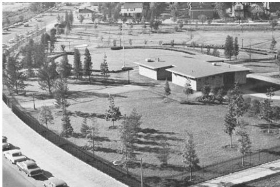
Aerial perspectives of recently completed path system, Administration Building, and garden improvements from 1964. New York World's Fair 1964-1965 Corporation, Post Fair Plan Queens Zoological and Botanical Gardens.
