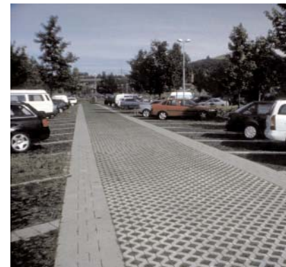
A parking garden pavement detail. Photo courtesy of Conservation Design Forum.
