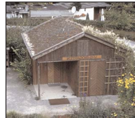
A green roof on a garden shed. Photo courtesy of Conservation Design Forum.
