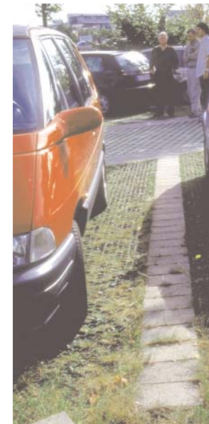
A parking garden pavement detail. Photo courtesy of Conservation Design Forum.
