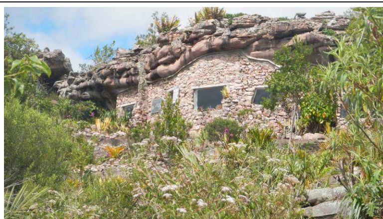
Built under a rock ledge, this former miner's hut has been repurposed as the Mucugé municipal park's visitor center.
