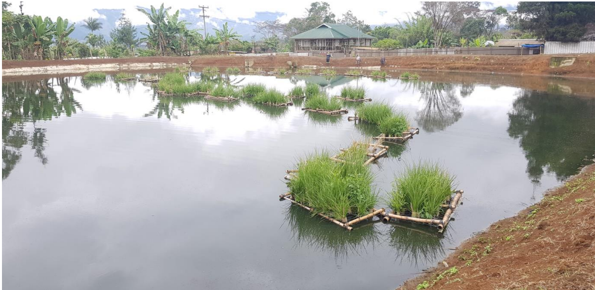
Picture 7: Sewage effluent treatment in 2019 (Goroka, Papua New Guinea)
