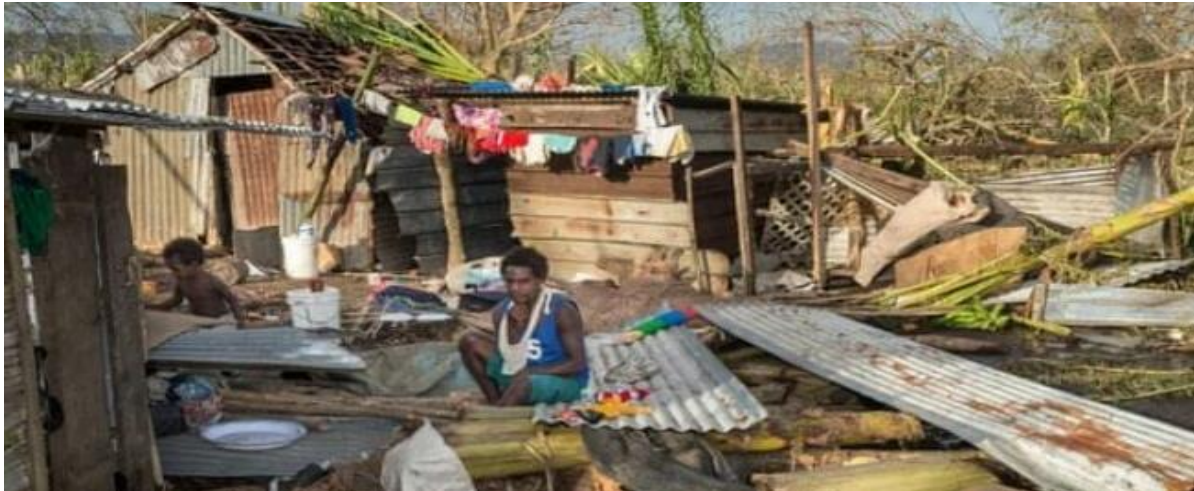
Picture 42: A villager in front of his damaged home (Port Vila, Vanuatu) – Picture by J Robertson
