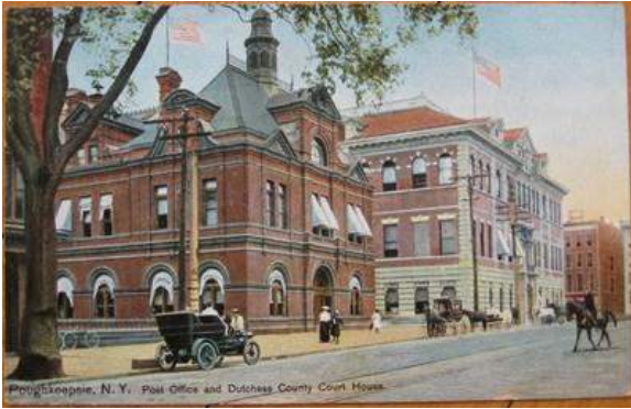
1902-1903 (present) Courthouse at right
