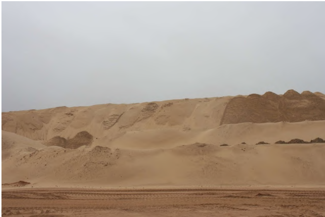
Plate 1 Mine Pit Undergoing Backfilling (Hose Mine)
