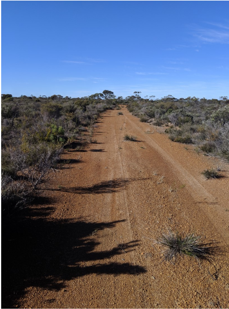
Figure 11. Completely Degraded Condition: Photo showing track which has not been rehabilitated, this track and other similar tracks could be easily rehabilitated, unless they are kept for fire or management access. Photo taken at GDA 94 Zone 51 386945.3M S 6284348.9M N Facing East.
