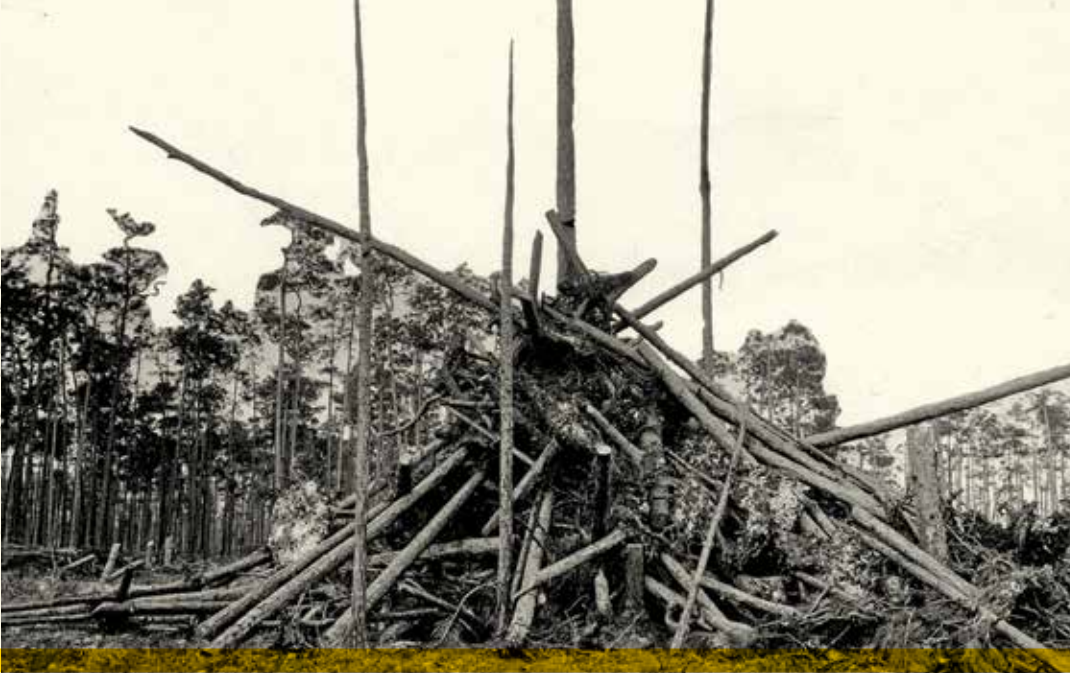
LEFT Pinelands near Hattie Bauer hammock, Dade County. Clearing land. Pine trees pulled out by the roots and piled up for burning! January, 1916. Photo by J. K. Small.
