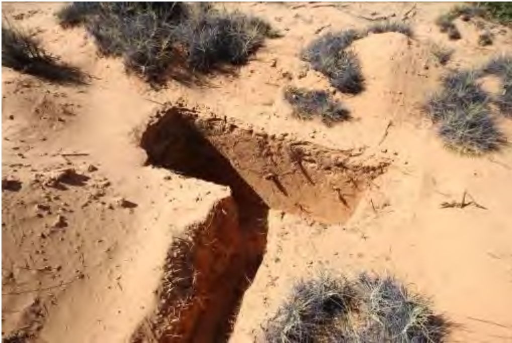
Figure 15. Trench (note: vertical wall in background and fauna escape ramp in foreground).
