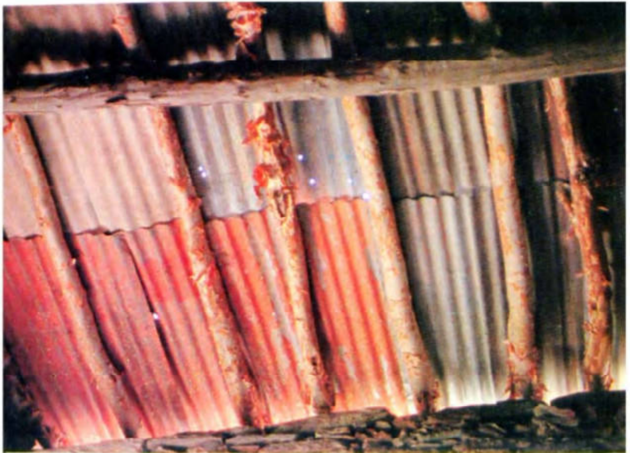
Betula logs : used in roof making
