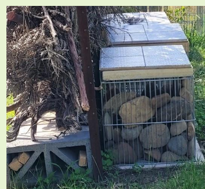
Besser blocks and rock gabions.
