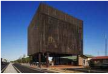
Barcaldine Tree of Knowledge<, J.W. Wilson Award for Building of the Year Central Queensland, Brian Hooper Architect and m3architecture. Photo by Jon Linkins. Image courtesy of Australian Institute of Architects.
