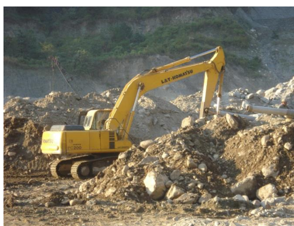
J: Construction of motorable road.
