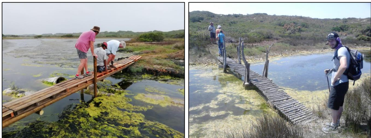
Figure 2.21 Low-impact walkways across watercourses to support nature-based recreation in the Kabeljous Nature Reserve.
