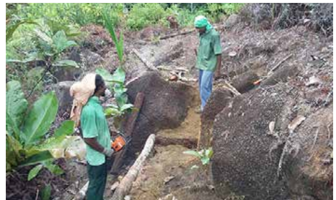
Construction of the nature trail (J Mougale)
