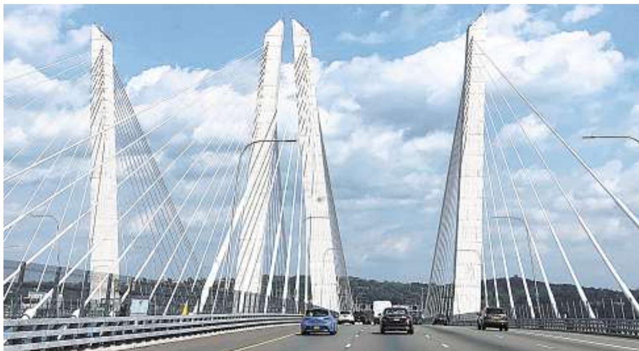
The New York State Thruway Authority has spent about $3.7 billion to build the Mario M. Cuomo Bridge, which fully opened in 2018.
