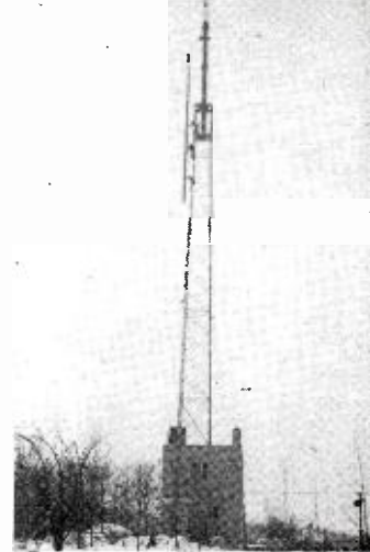
RIGGERS place 6-bat-wing RCA antennae atop tower high in Watchung Mountains in New Jersey as preparations for opening of WATV, state's first video station, at Newark on Channel 13 (210-216 mc). Permittee is Bremer Broadcasting Corp.
