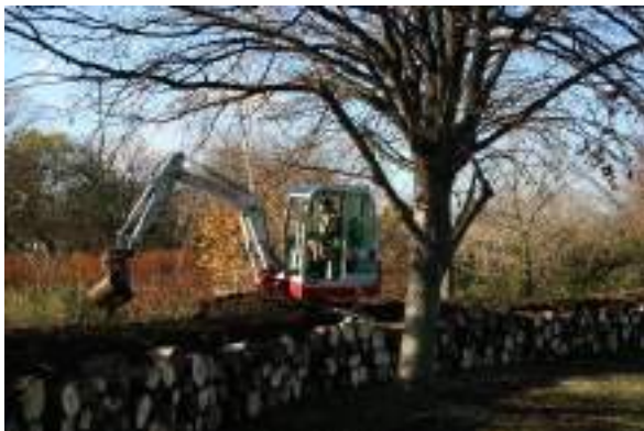
Example of hibernacula created using site won woody material
