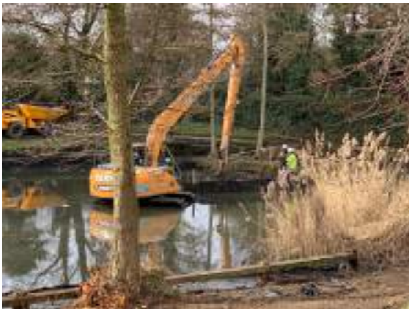
De-silting and boardwalk construction
