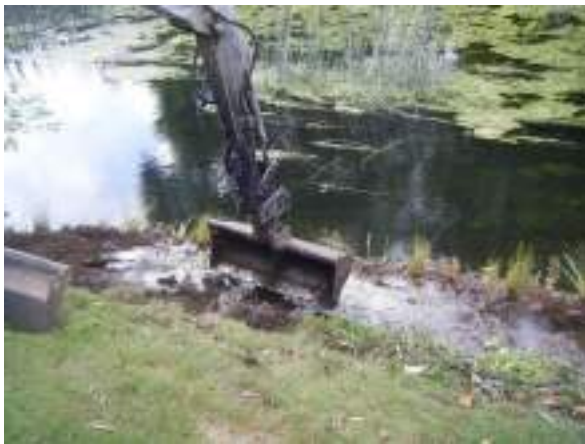
Shallow marginal habitat under construction
