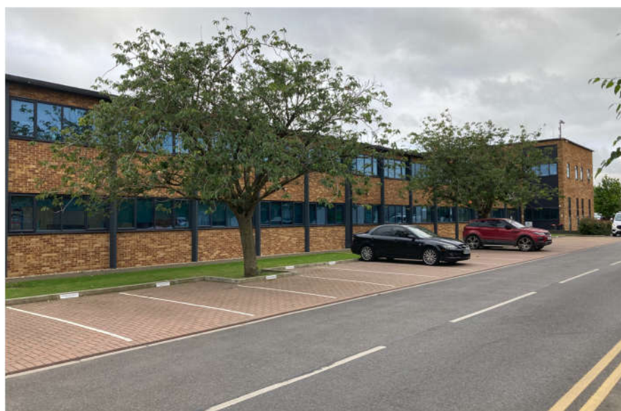
Figure 20. Boston House on Grove Business Park, home to many start-up companies.
