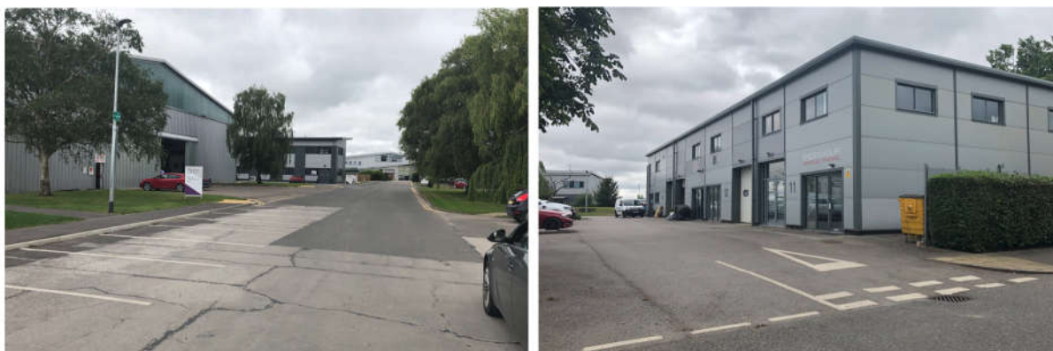
Figure 45. Grove Business Park
