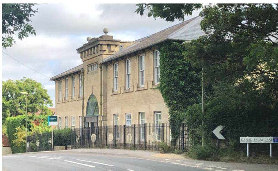
Figure 38. Listed building. The former 19 th century Nalder Manufacturing centre.
