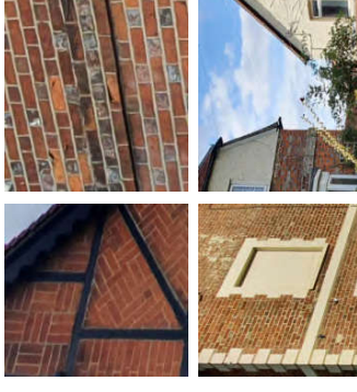
Timber frame with herringbone brick infill - decorative infill brick appears commonly in the wider area and even on later modern buildings to add interest.
