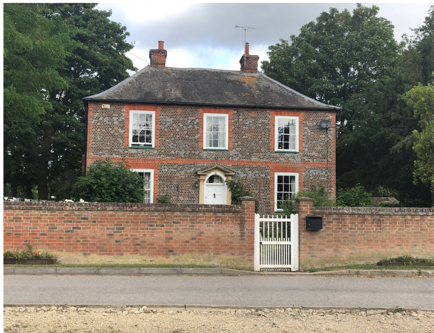
Figure 37. Listed building 18 th century farmhouse.
