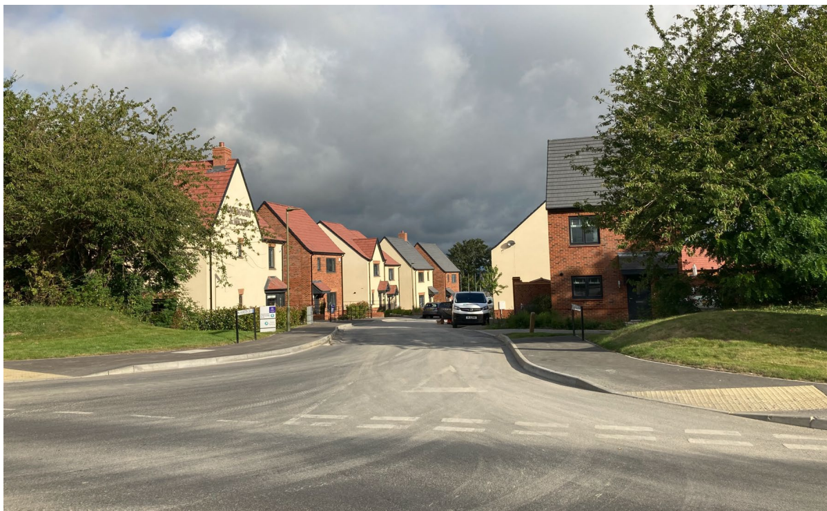
Figure 16. The new Childrey Park development on the A417.
