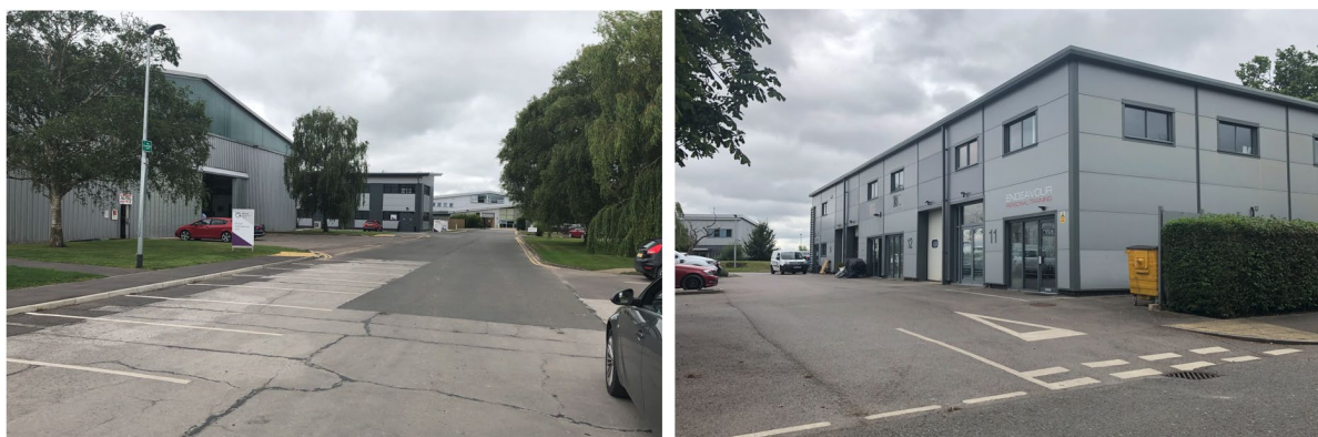
Figure 45. Grove Business Park
