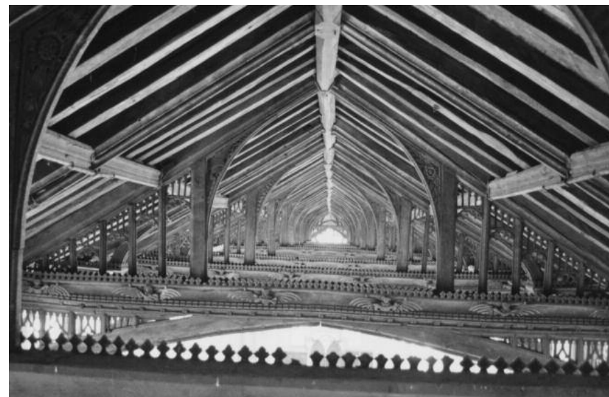
A view through the tie-beams in the roof
