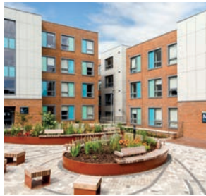
Hiatt Baker Hall North Residential Village Undergraduate residence 747 places Catered and self-catered 2.2 miles to campus From £152 per week
