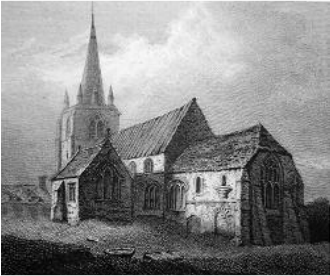
Figure 12 St Mary's before the 1829 restoration
