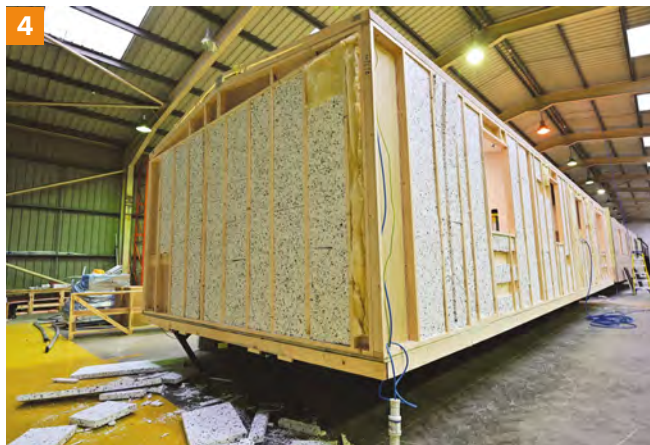
1 By the 1960s, statics were growing in width, from 7ft 6in to 9ft 6in 2 The holiday home was often confused with the caravan, but it's an entirely different construction, as this 1968 twin unit shows 3 Unlike statics, holiday homes are a much more permanent structure 4 Static caravans are fully insulated throughout, including the floors
