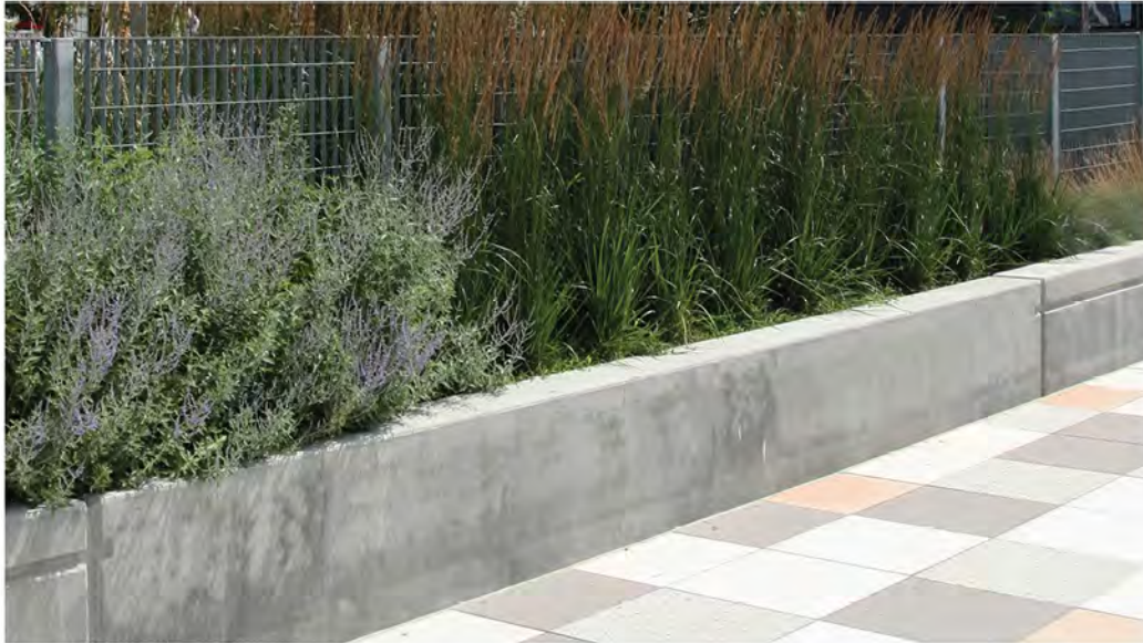
WALLS: Poured in Place Concrete
