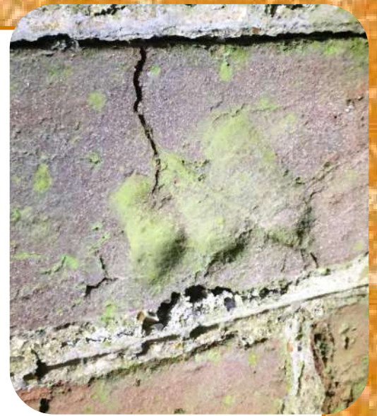
Fingerprint marks in the brickwork of Stratton's Tower indicate that they were hand made, and likely Tudor in origin
