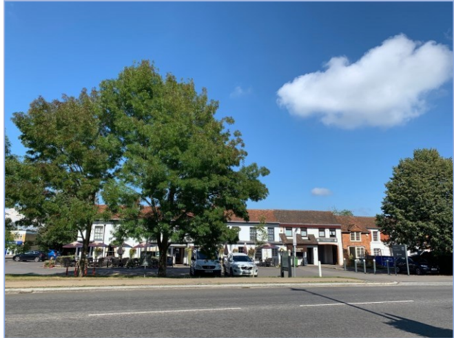
Saddlers Court, Reading Road, Yateley
