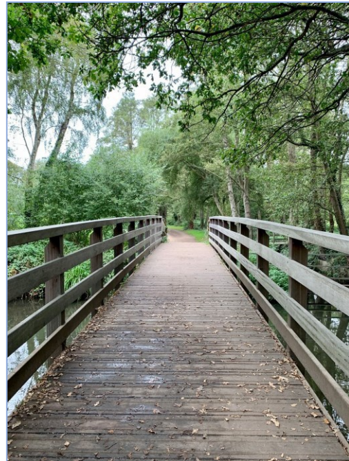
Bridge over the River Blackwater Photo courtesy of Kirsty Daws
