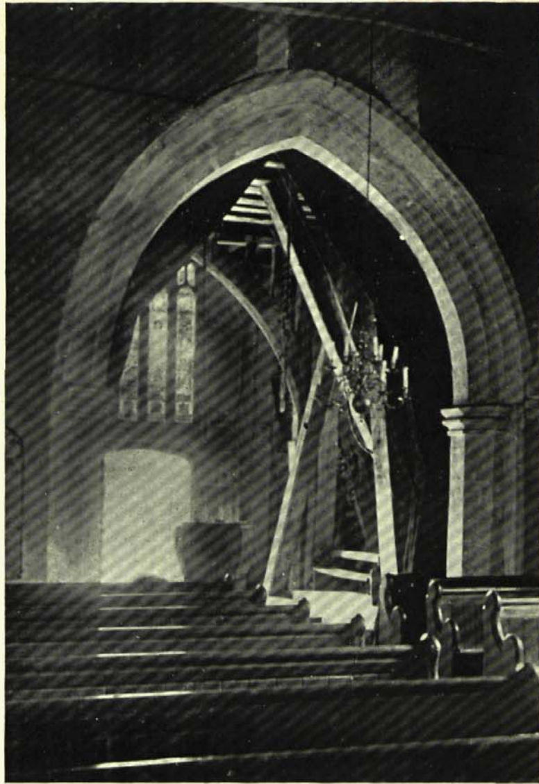
Arch of Tower, Yateley Church.
