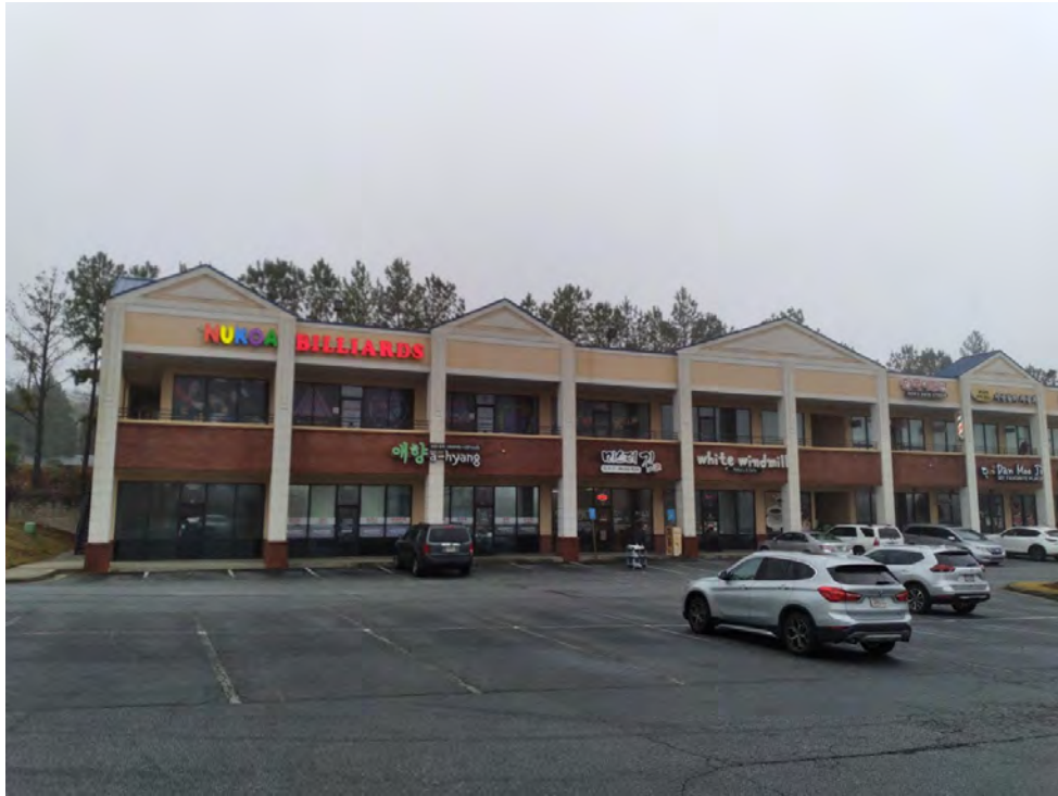
WEST END OF EXISTING BUILDING
