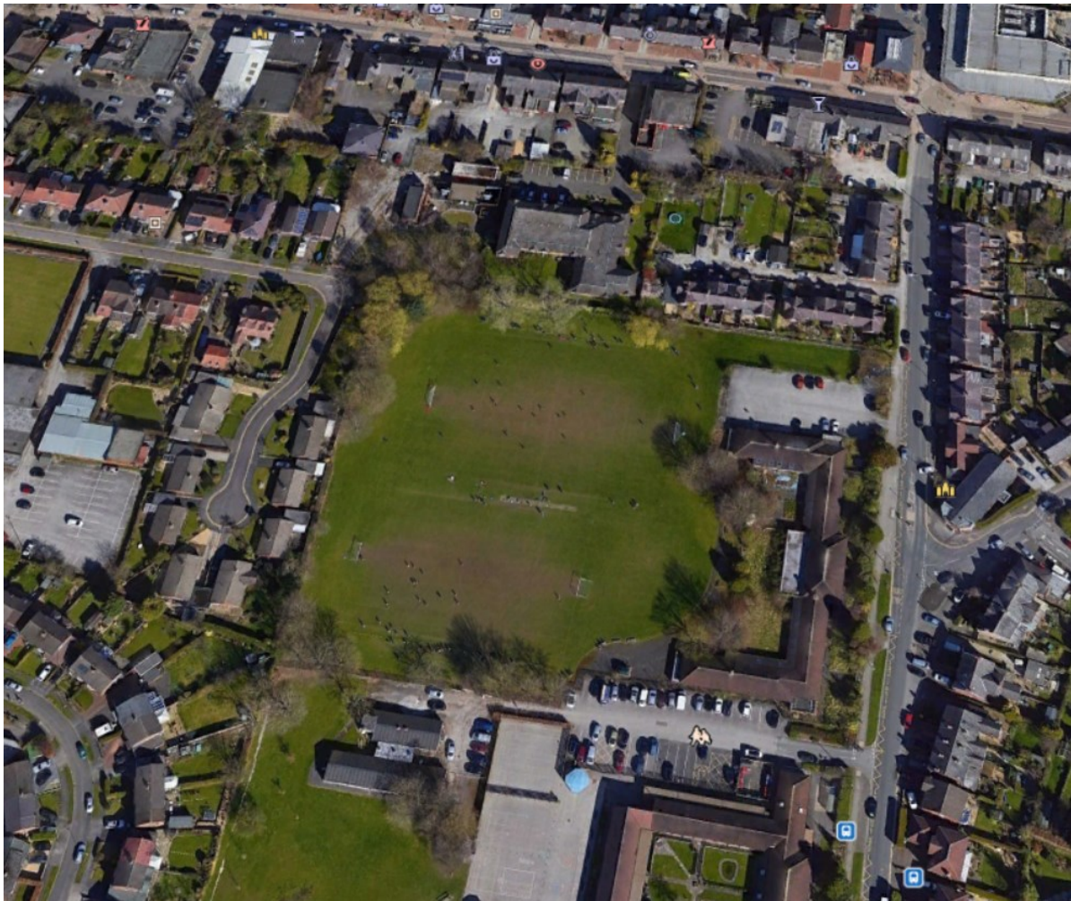
Figure 3.7: Overview of Former Vernon Infants School
