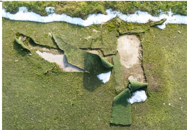
Figure 3: Artificial cricket wicket shows significant damage to the carpet and is suffering with excessive moss ingress.
