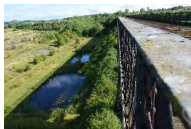
Bennerley Viaduct east to Awsworth
