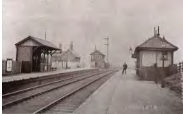
Awsworth Station 1909 (RM)
