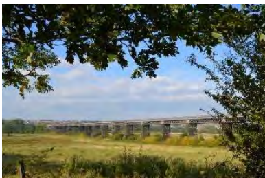
Bennerley Viaduct west to Ilkeston
