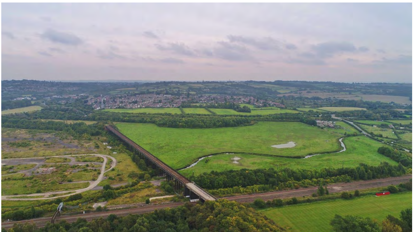
Awsworth Parish from the West – Photo by Paul Atherley Back Cover – Aerial Views of Awsworth Village looking East - Photos by Paul Atherley
