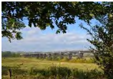
Bennerley Viaduct Grade II*
