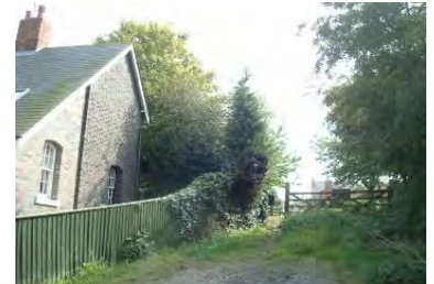
Site of level crossing at station
