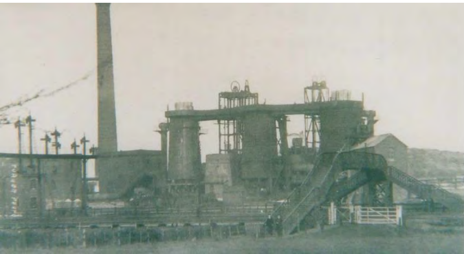
Bennerley Blast Furnaces 1910 (RM)
