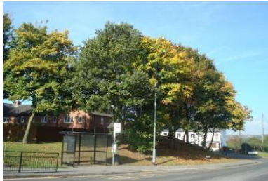
Embankment at Gin Close Way
