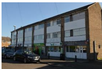
Lawrence Avenue Shops
