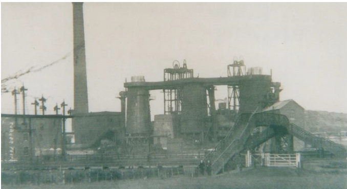
Bennerley Blast Furnaces 1910 (RM)
