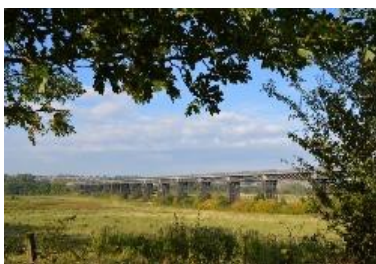
Bennerley Viaduct Grade II*
