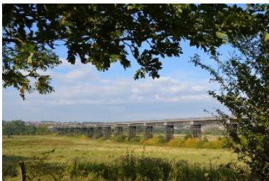
Bennerley Viaduct west to Ilkeston
