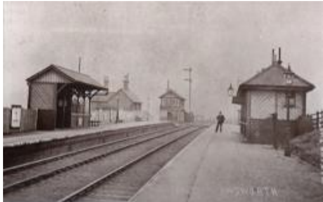
Awsworth Station 1909 (RM)
