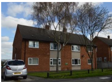
Main Street Flats
