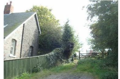
Site of level crossing at station
