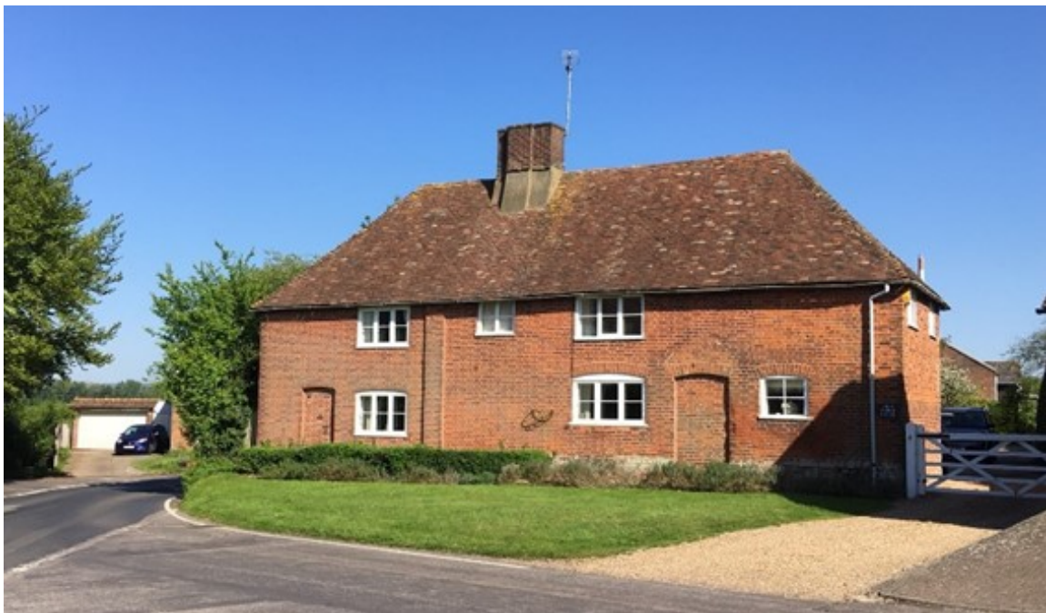
Old Forge House, The Lees
