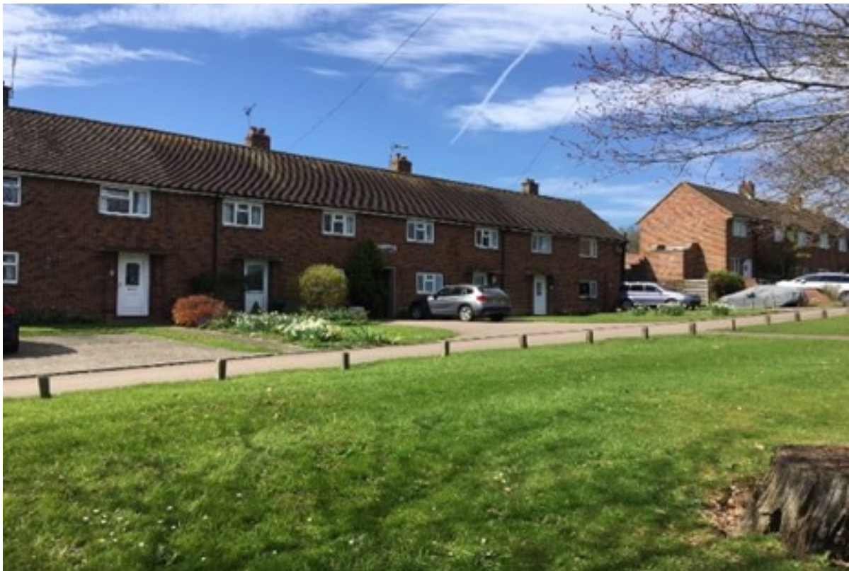
Middleton Cottages, Faversham Road
