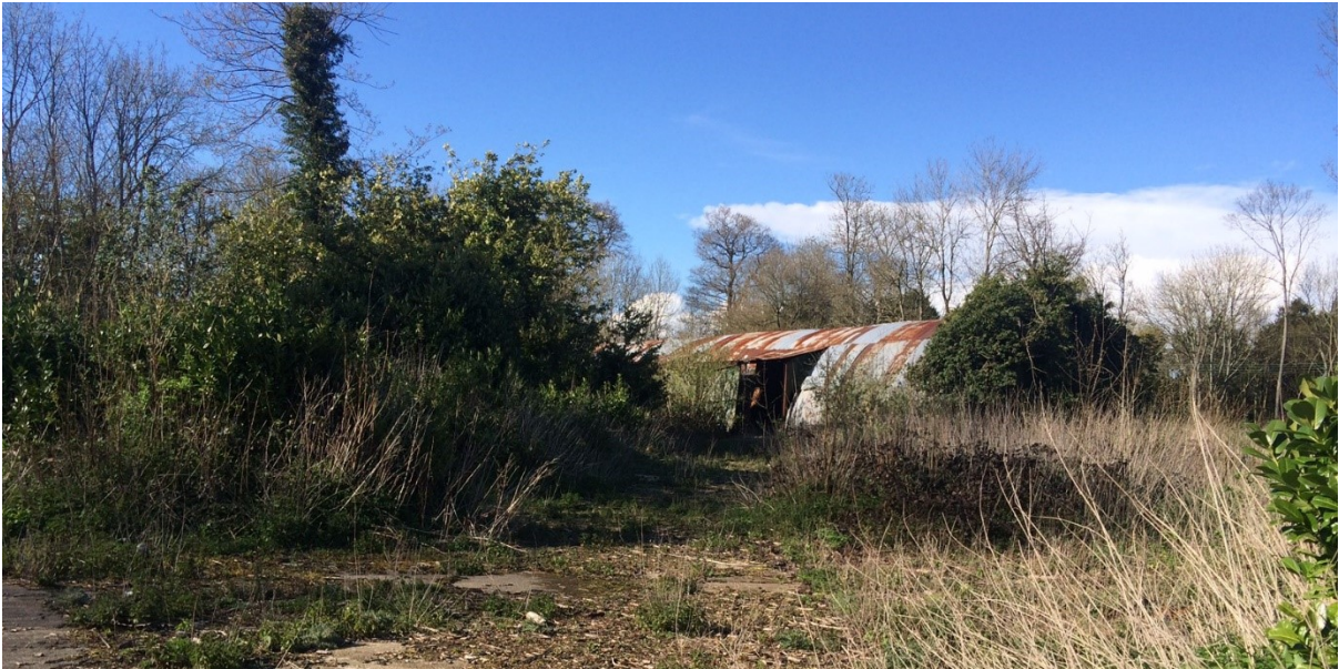
Rook Toll, Faversham Road
