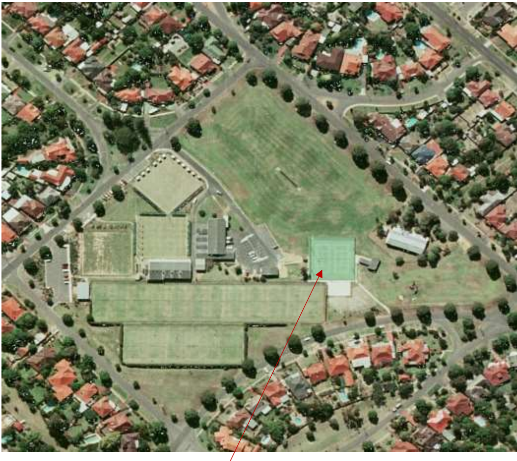
19 June 1985- Two hard courts completed and road way closed
