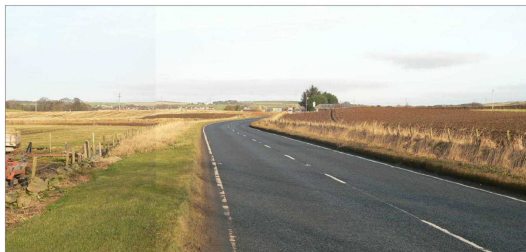
4. View north along the A947 near Kinmundy, Newmachar barely visible in centre distance
