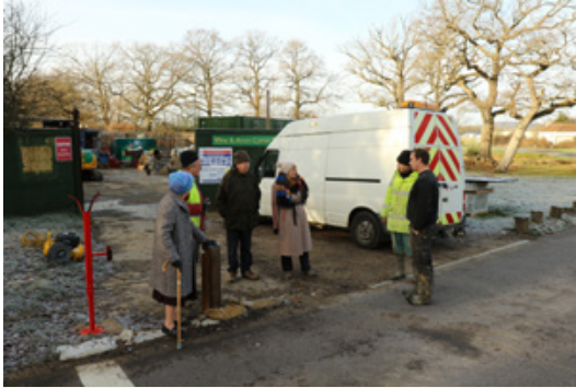
27th December 2016: An informal site conference outside the Compasses compound.
