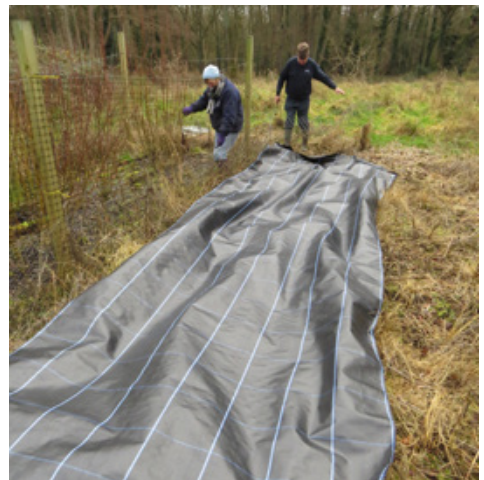
Preparing the ground for the extended osier bed in Hunt Park.
