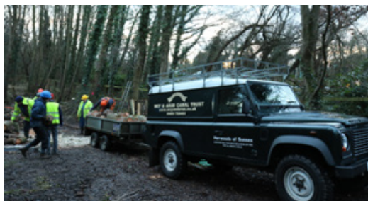
The Trust's Land Rover in use for clearing the Hunt Nature Park works compound.
